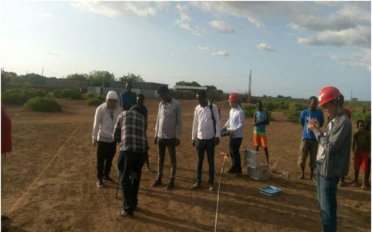
Figure: photo taken from camera at site
